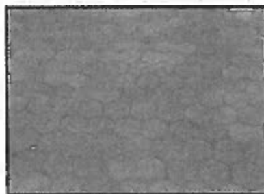
Good paved surface without issues
